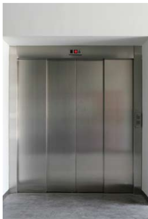
4-panel central opening AUTOMATIC VVVF door
